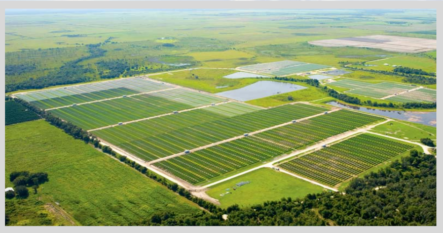
At 25 MW peak output, the DeSoto Next Generation Solar Energy Center in DeSoto County Florida is currently the largest PV installation in the United States. The facility came online in 2009 and generates over 42,000 megawatt-hours of electricity each year. (Photo—Florida Power & Light)
