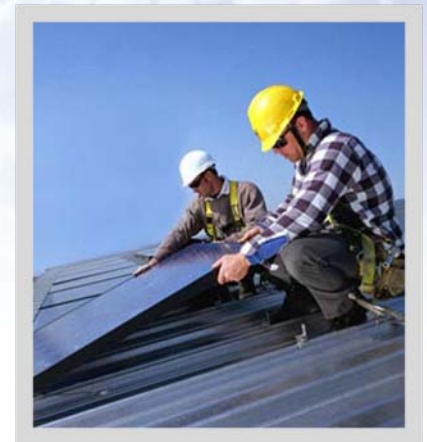
Solar installation workers mount PV panels on a private home. These panels generate clean, pollution-free electricity and can reduce or eliminate monthly electricity bills. In 2008, over 16,000 residential systems were installed, with an average size of just under 5 kilowatts (kW). (Photo – NREL)
