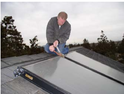
An installer mounts a solar water heater flush to the roof.
