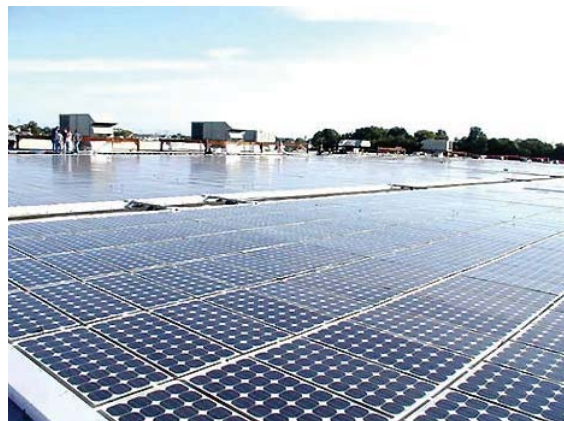
Source for facts and photo: Long Island Power Authority
