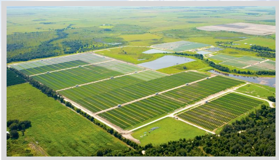
At 25 MW peak output, the DeSoto Next Generation Solar Energy Center in DeSoto County Florida is currently the largest PV installation in the United States. The facility came online in 2009 and generates over 42,000 megawatt-hours of electricity each year. (Photo—Florida Power & Light)
