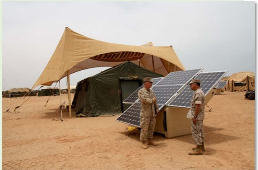
Operational PV system. For more information, visit www.thezerobase.com (Photo: ZeroBase Energy, LLC)
