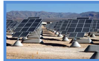
Project Name: Nellis Air Force Base Developer: MMA Renewable Ventures Electricity Purchaser: Nellis Air Force Base Location: Clark County, Nev. Technology: PV Capacity: 14 MW Source: MMA Renewable Ventures
