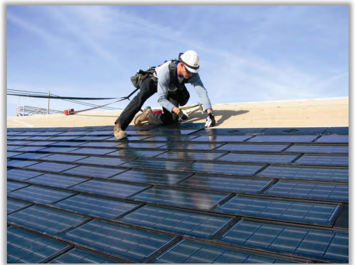
Worker installs solar shingles. (Dow Solar Solutions)
