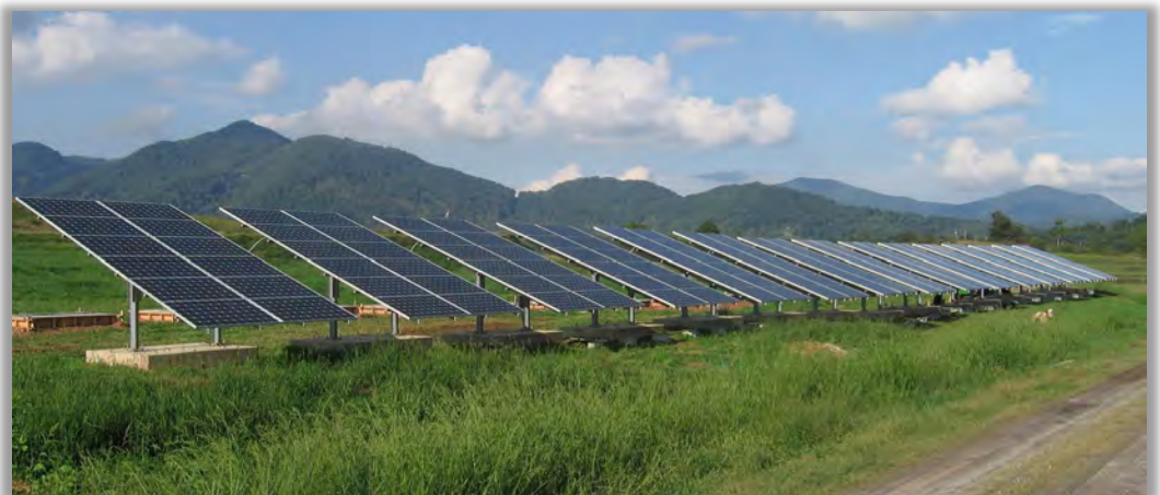
A 555-kW PV system on landfill in Canton, North Carolina. (Joanna Malcolm, FLS Energy; Suniva)
